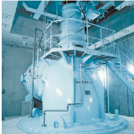
Dewatering pump with adjustable vane (Size:2,400mm, Driver:1,103kW)
