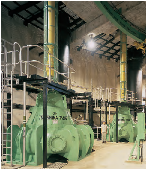
φ 1300 Vertical end suction sewage pumps (HARBOUR AREA TREATMENT SCHEME, HONG KONG)
