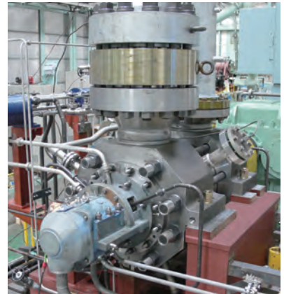
HP Ring section boiler feed pump (RABIGH ARABIAN WATER AND ELECTRICITY, SAUDI ARABIA)
