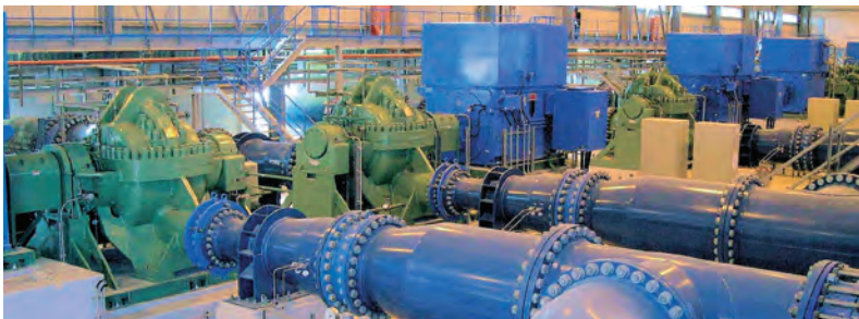
φ 800 x φ 500 double suction drinking water transmitting pumps with high total head 250m (SHUWEIHAT WATER TRANSMISSION SCHEME, U.A.E.)
