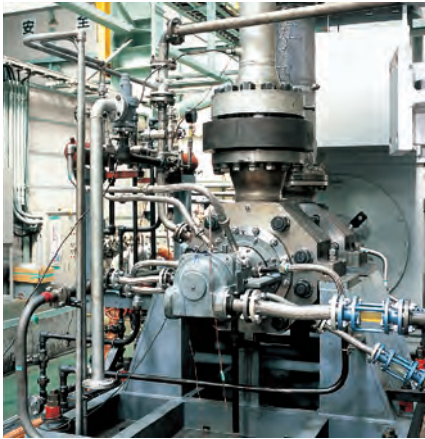
Ring section boiler feed pump for combined cycle power plant (FUJAIRAH WATER AND POWER PLANT, U.A.E.)
