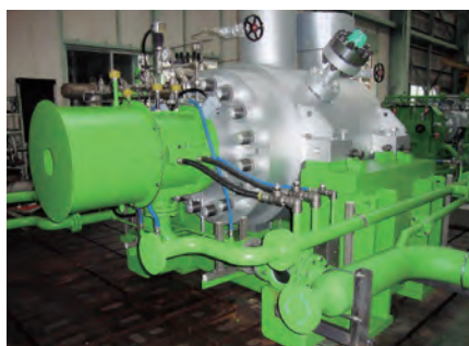
φ 300 Boiler feedwater pump (CIREBON COAL FIRED POWER PLANT, INDONESIA)
