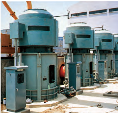
φ 1000 Sea water pumps for LNG vaporizing plant (KOREA GAS CORPORATION, KOREA)
