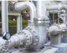
FEDCO's turbocharger for seawater desalination plant in Saudi Arabia
